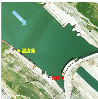
图2 溪洛渡坝前光纤、温度链位置 Fig.2 The location of optical fiber and temperature chain in front of Xiluodu dam
